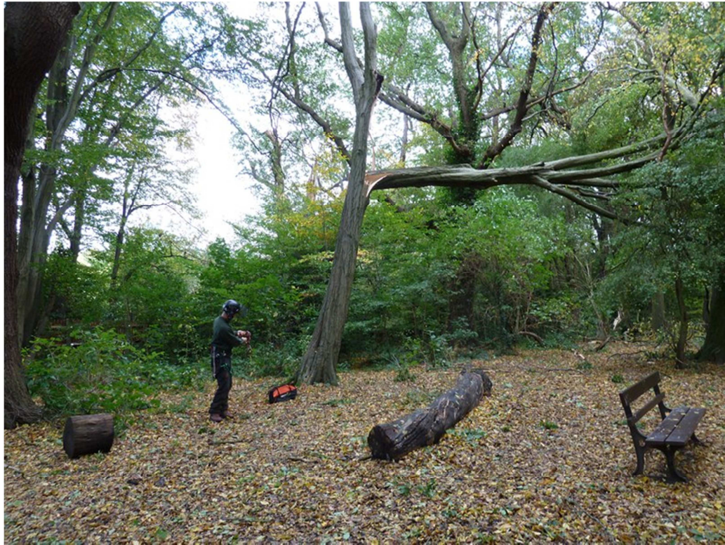
Figure 1: clearing storm damage operation
